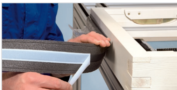
Sample installation (1-BT): Fitting wooden windows
