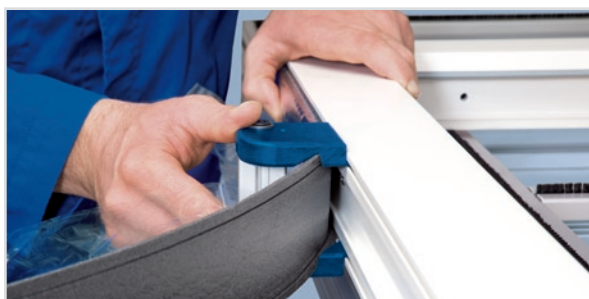
Sample installation (CB): Fitting PVC windows
